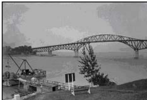
The old "Crown Point Bridge before it was demolished
