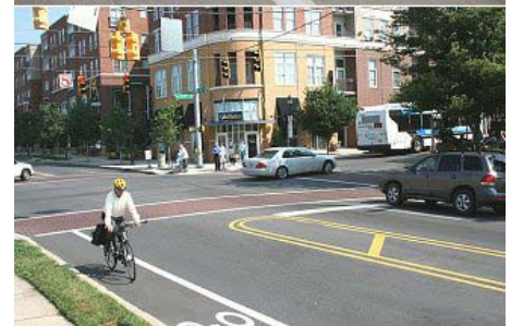
Different facilities for different roads. Right: a rural and an urban setting call for different types of complete streets treatments
